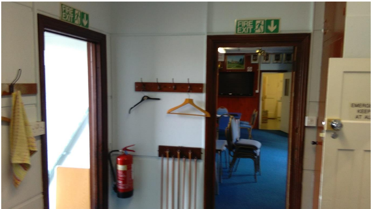
Existing changing area and partition wall view.
